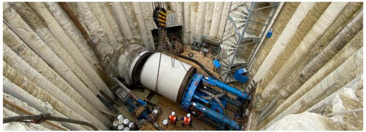
In the densely populated city of Gagny, just outside Paris, a large water collector was built by the use of microtunneling. This basin will serve as a rain collector, avoiding floodings in the event of heavy and long rain periods.
